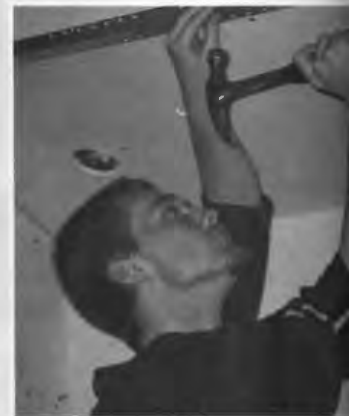
Senior Sean Dieter hammers into the drywall.
