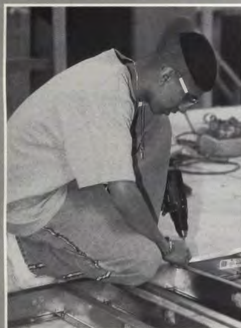
Abad Rubio works on an internal wall for an addition to the TCD building. Students in the Construction Trades classes were responsible for much of the work on the addition.
