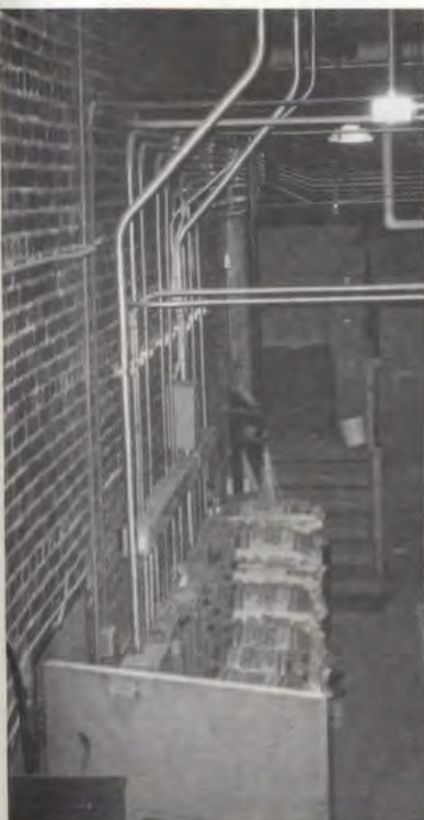
The basement of our school.
